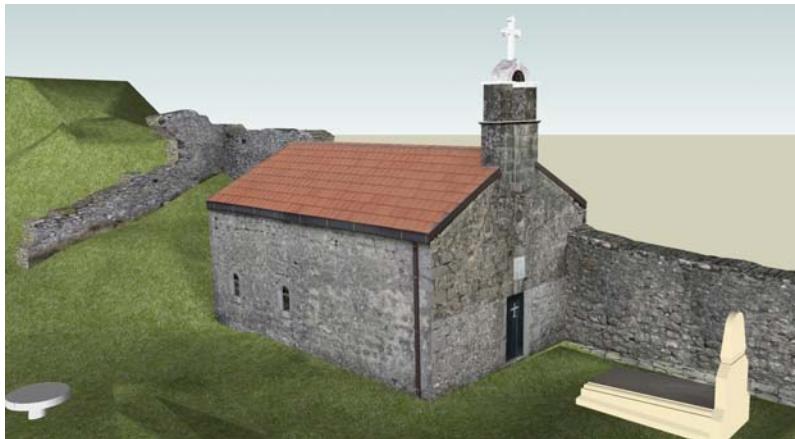
Picture 4. 3D model of the church at Medun (near Podgorica) generated from the data from laser scanning and digital photogrammetry
